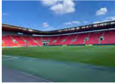
In Sep, 2021, our ENELTEC LED Stadium Lights were being installed in the Biggest soccer field in Czech . According to our dialux simulation , the Average lux , Uniformity , and GR , all have reached and even surpassed the UEFA illuminance level A.
